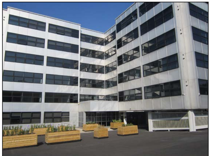
Bovis House, 142 Northolt Road, South Harrow
