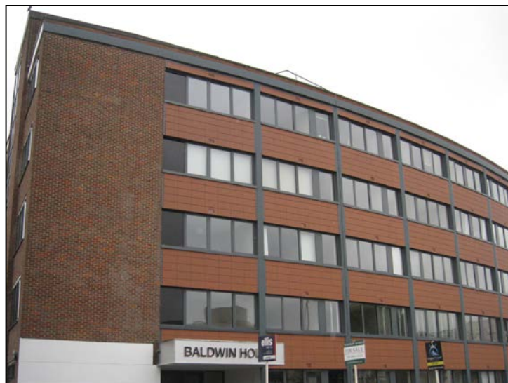
Baldwin House, 2 Gayton Road, Harrow
